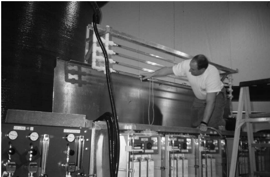
Fig. 7. Quartz sleeves are cleaned on an open channel UV system (with low pressure/low intensity bulbs) at the Freshwater Institute.
